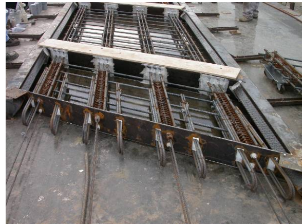
Figure 4. Longitudinal joint reinforcing
