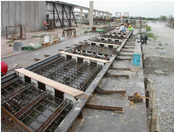
Figure 1. Panel forms and reinforcing
