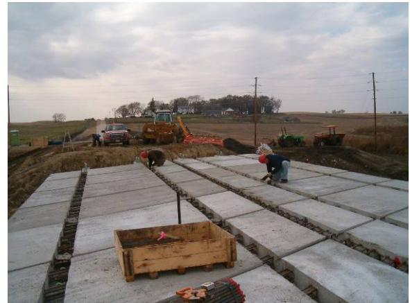
Figure 8. Leveling device installation
