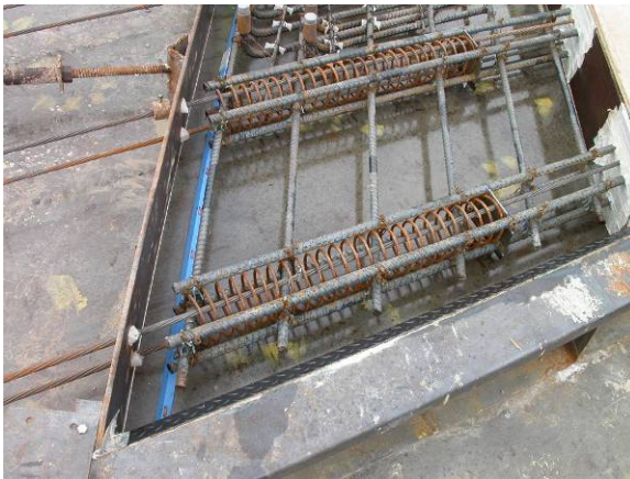
Figure 3. Spiral reinforcing
