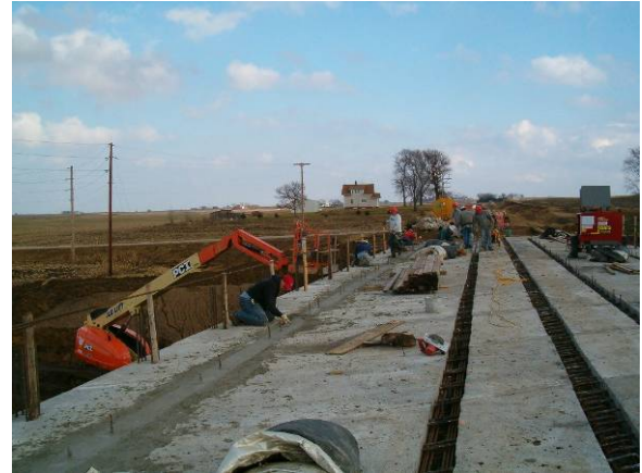
Figure 10. Casting longitudinal joints
