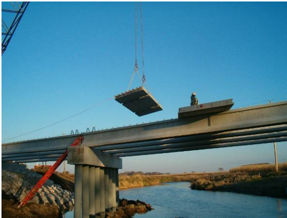
Figure 7. Deck panel erection
