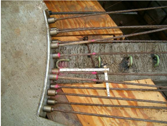
Figure 9. Strand elongation check
