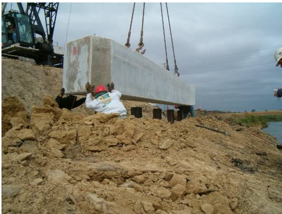
Figure 5. Setting precast abutment
